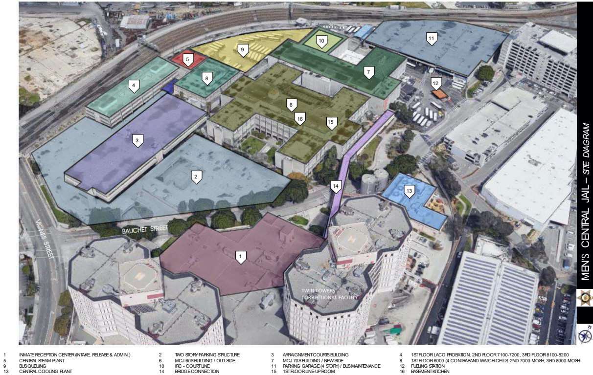
Figure 2. Arial View of MCJ Complex
